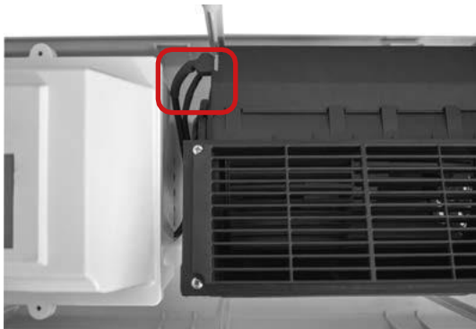
Fig. 7.4.2.6: Connecting the fan plug
