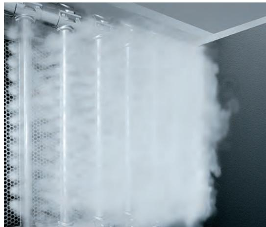
The hot dry steam is absorbed quickly and uniformly by the air stream.
